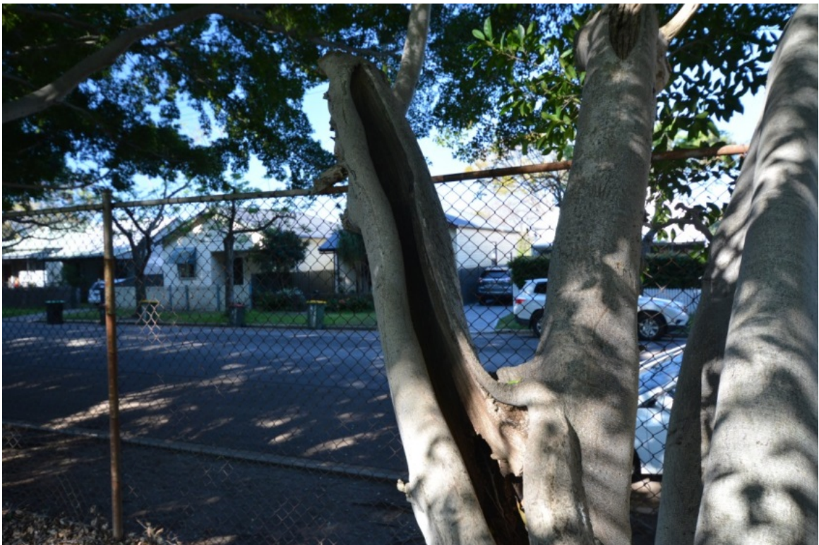
FIGURE 10: ONE OF THE WORSE EXAMPLES OF DECAY ORIGINATING FROM THE PREVIOUS REMOVAL OF AN OVERHANG BRANCH.
